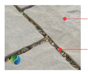
The pavers used in a permeable installation look very similar to traditional pavers, but are made with extra space between them so rainwater can flow back into the earth below, instead of running off the surface into storm sewers.
