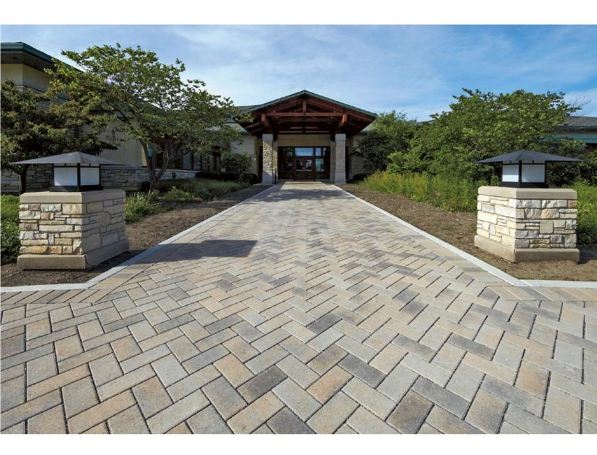
**USING PERMEABLE PAVING** for residential driveways and streetscapes not only allows builders to increase the size of the impermeable building footprint, but it also reduces the cost of stormwater management infrastructure.
