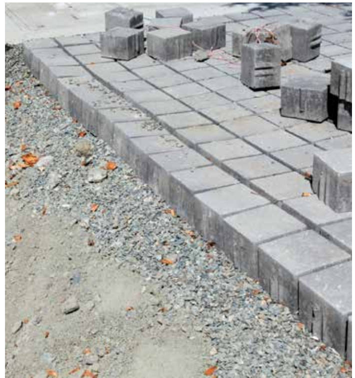
Pavers pulled for underground repair
