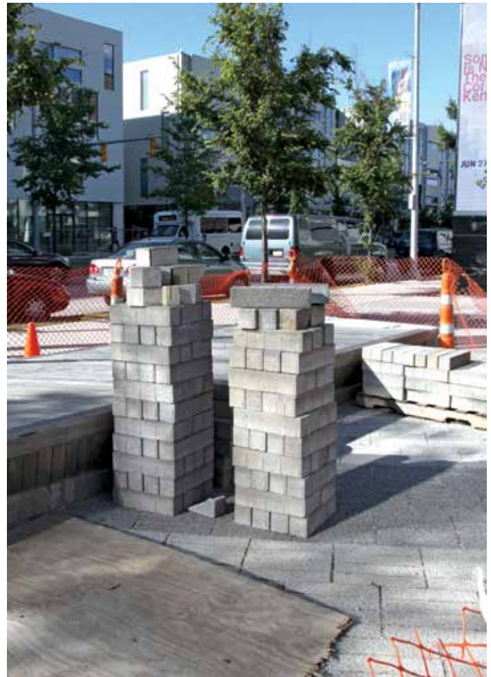
Site repair awaiting reinstatement
