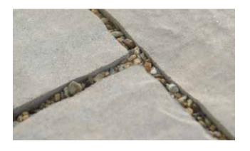
Special materials are used in the joints and in the permeable base below, to encourage water to flow through.
