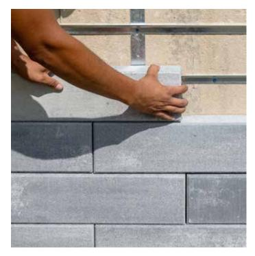
The U-Cara Wall Mount System allows project by cladding existing structures like unsightly exposed foundation areas or concrete steps with U-Cara fascia panels.
